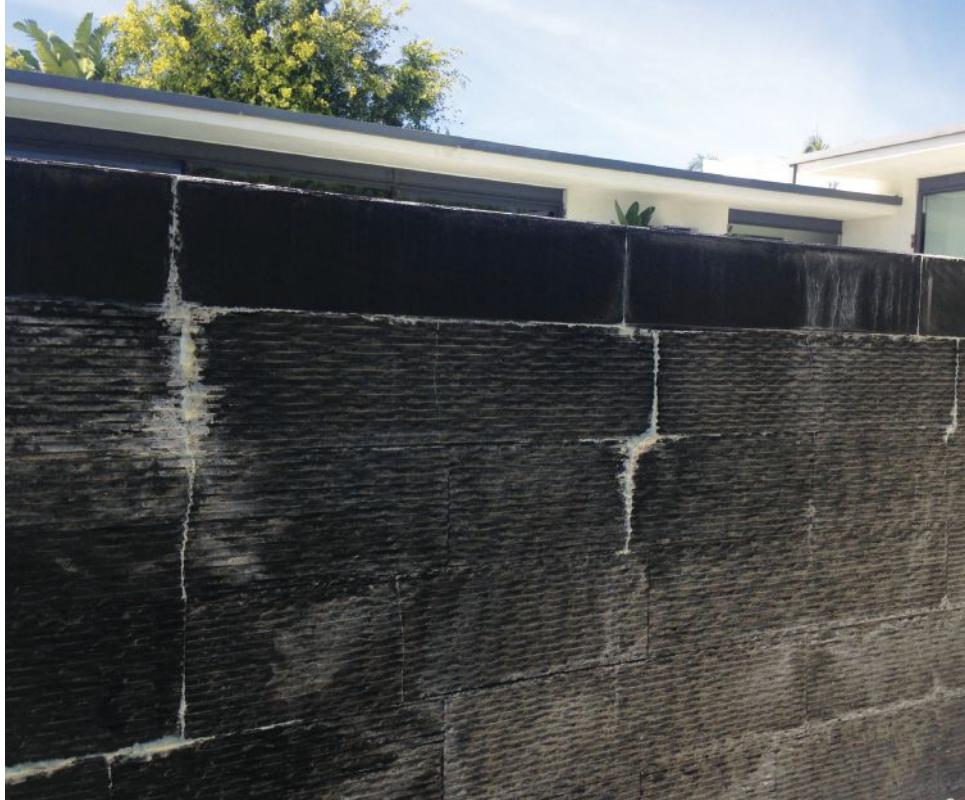
On these stone-tile installations that National Tile and Stone Authority inspected, latex has re-emulsified through the grout, likely due to inadequate curing times for the thinset.
