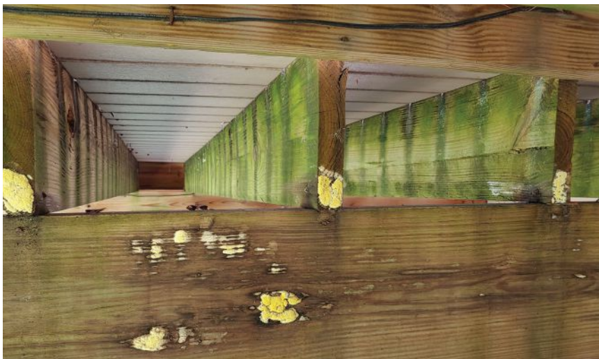
Advanced decay of joists and beam treated to “Above Ground” based on an available treatment tag. The tag did not indicate an AWPA Use Category System.
