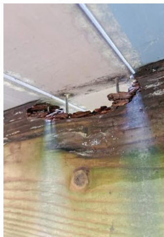
Advanced decay of joists and beam treated to “Above Ground” based on an available treatment tag. The tag did not indicate an AWPA Use Category System.
