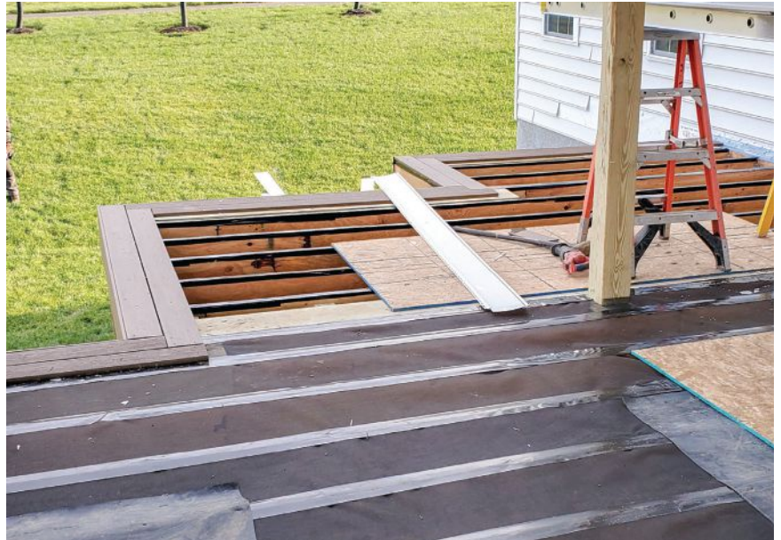
The PWT preservative-treated LVL framing has been flashed for additional protection.
