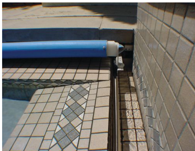
On vanishing edges, automatic-cover tracking is placed at the top of the wall, elevated slightly off the surface to form a gap for water to flow through.
