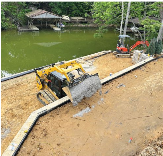
Left: After the pool was in place, workers began the process of building the retaining walls and backfilling them with gravel and soil to create the two lower terraced levels. Right: Here, the crew is installing the stone steps that connect the lowest tier to the dock system.
