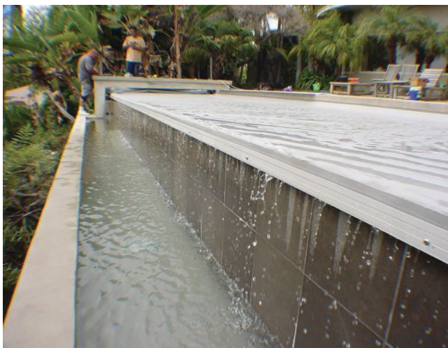
On vanishing edges, automatic-cover tracking is placed at the top of the wall, elevated slightly off the surface to form a gap for water to flow through.
