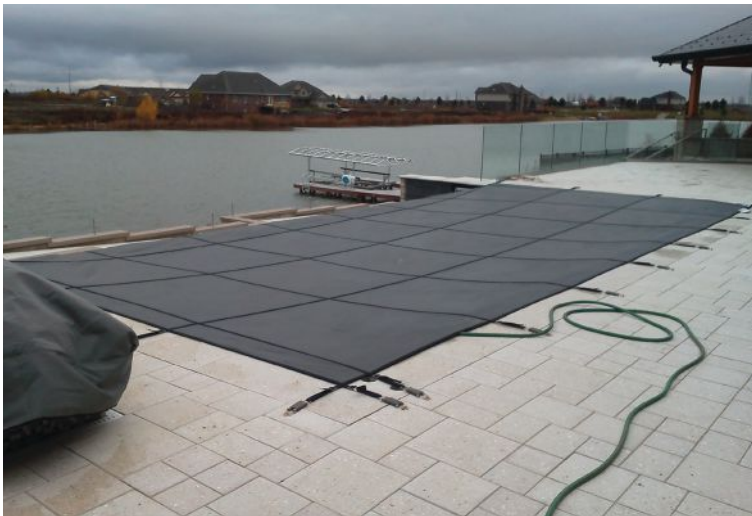
The mesh safety cover straps are secured to the vanishing-edge catch basin.
