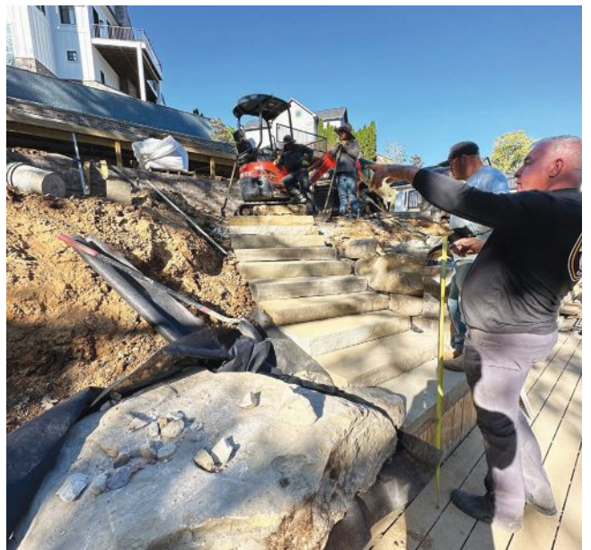
Left: After the pool was in place, workers began the process of building the retaining walls and backfilling them with gravel and soil to create the two lower terraced levels. Right: Here, the crew is installing the stone steps that connect the lowest tier to the dock system.
