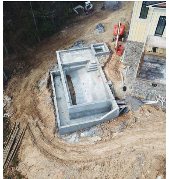
Left: Site work began while the house was still under construction. Right: Early in the project, workers formed and poured the infinity edge pool.
