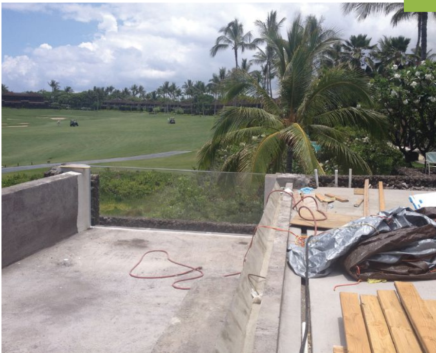
Acrylic expands and contracts more than concrete. Experts generally recommend flexible caulks, grouts and membranes so the panel can move. In the case of vanishing edges, the hydraulic system should probably allow for more water in transit so flows can be adjusted as the wall expands up.
