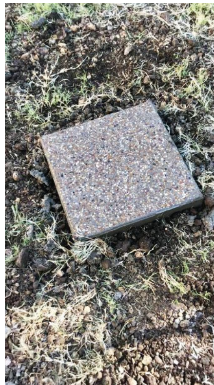
The pergola's support posts bear on the concrete patio and on 16-by-16-inch piers with a washed aggregate finish.
