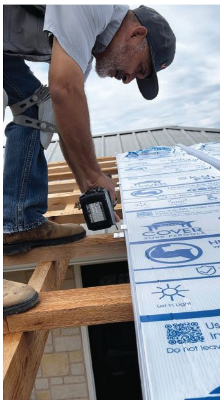
The panels are installed starting at the center and working towards both ends. They are fastened to the purlins with special metal clips.
