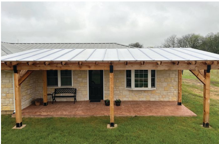
The outside edge of the last panel is cut to fit, then covered with a metal U-edge profile that is screwed to the purlins (right).
