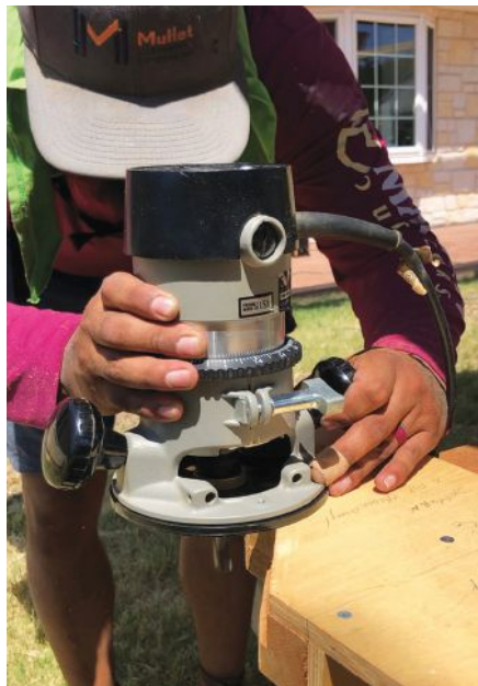
... and another one to shape the tails of the 2x6 rafters.
