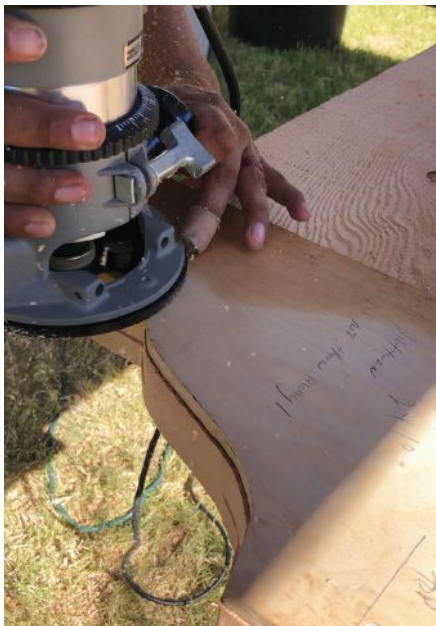
The author used one jig to shape the ends of the double 2x12 beams ...
