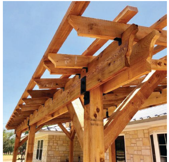
The pergola's support posts bear on the concrete patio and on 16-by-16-inch piers with a washed aggregate finish.
