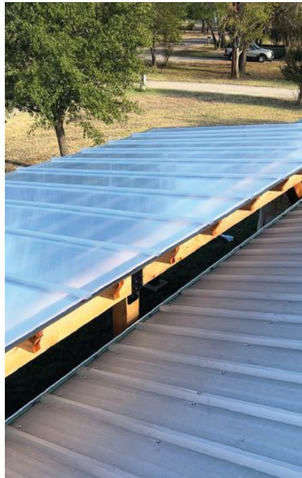
Raising the inner beam of the free-standing pergola above the eaves of the home's hipped roof allows for air circulation as well as the recommended slope (1 inch in 4 feet) for the polycarbonate roof panels.
