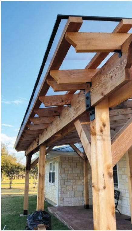
The outside edge of the last panel is cut to fit, then covered with a metal U-edge profile that is screwed to the purlins (right).
