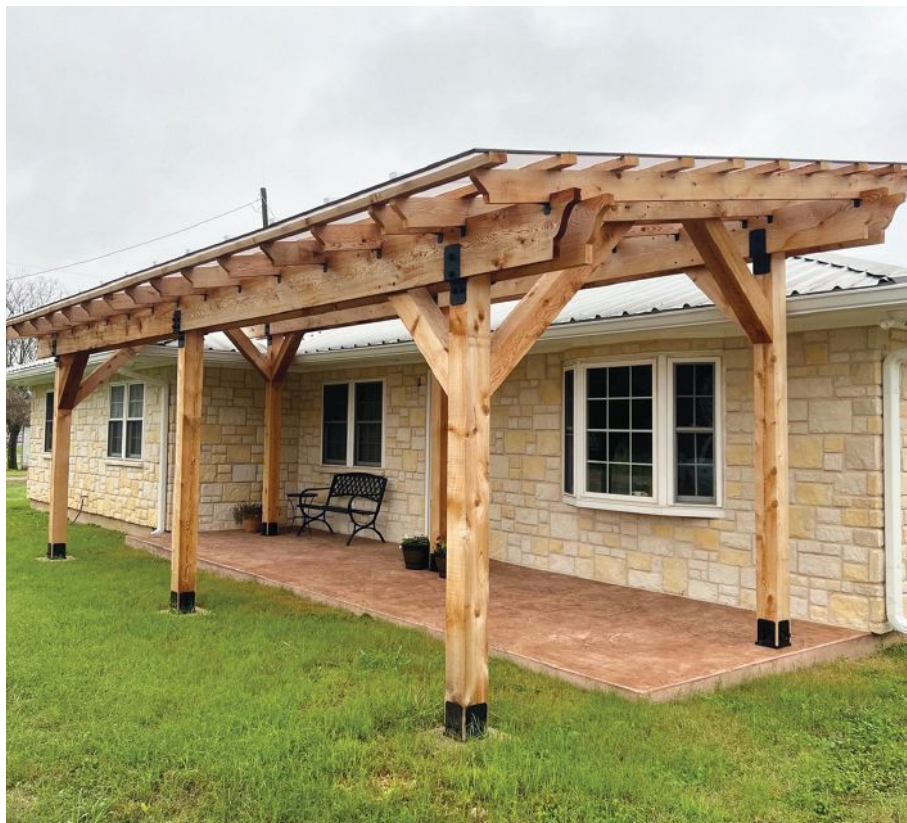
Framed as a freestanding pergola but with a clear roof, this patio cover is designed to allow plenty of light into the home.
