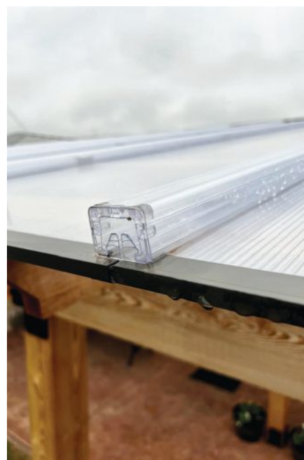
Friction-fit connector caps are tapped into place with a mallet to cover the raised seams between panels and prevent leakage, then plugged with matching end caps. The ends of the hollow panels are covered with a special vent tape followed by a flute cover, allowing for ventilation while blocking access to insects.
