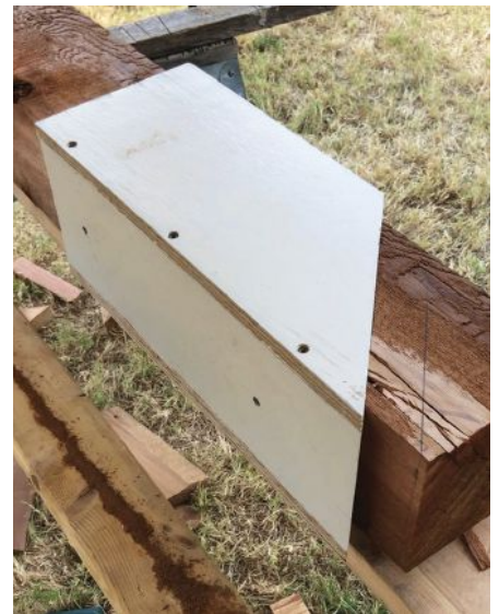
A simple guide made out of scrap material allowed the author to make the clean and accurate 45-degree-angle cuts needed for the diagonal braces that reinforce the post-to-beam connection.
