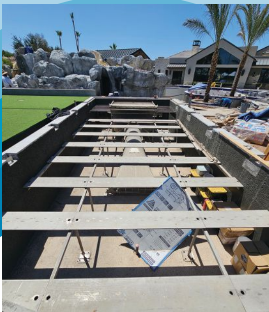
Pictured left: The surf simulator in progress. The inflatable portion will sit atop the slats, with the funnel intake underneath. The notches in the edges of the basin will accommodate rollers for the movable floor. Right: The movable floor during installation, with the artificial turf pad below.
