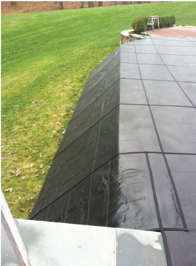
A safety cover extends over a vanishing-edge wall.
