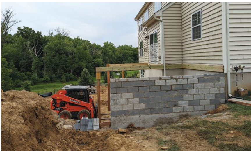
After the retaining wall was built, the author used his Kubota SSV65 skid loader to lift the heavy deck beam into position, so that the crew could begin framing the deck.
