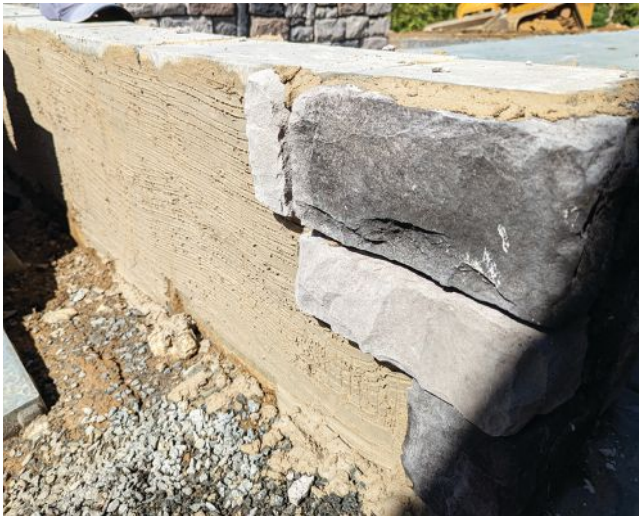
The block walls are finished with manufactured stone veneer.
