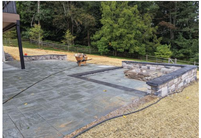
The sitting walls are capped with manufactured pavers that match the edging around the sunken fire pit. A layer of straw helps protect the newly graded and re-seeded lawn from erosion while the grass takes root.
