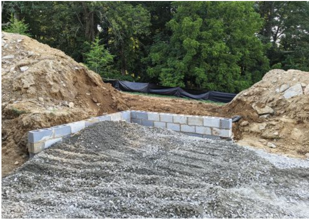
The block sitting walls at the corners of the cast-stone-paver patio are supported by full below-frostline footings.
