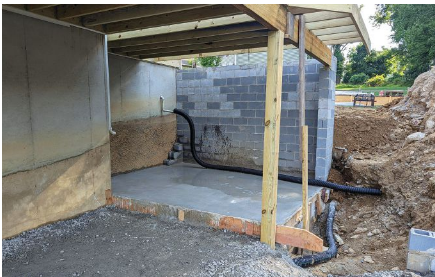
Workers poured the concrete slab floor for the storage room while the rest of the crew worked on the deck framing.
