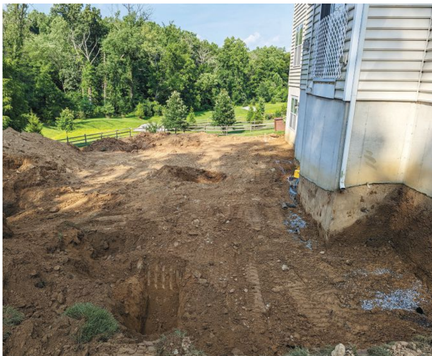
After the site was leveled, the author used his Kubota excavator to dig for the footings for the deck and storage-room walls, and for the sitting walls at the corners of the patio.
