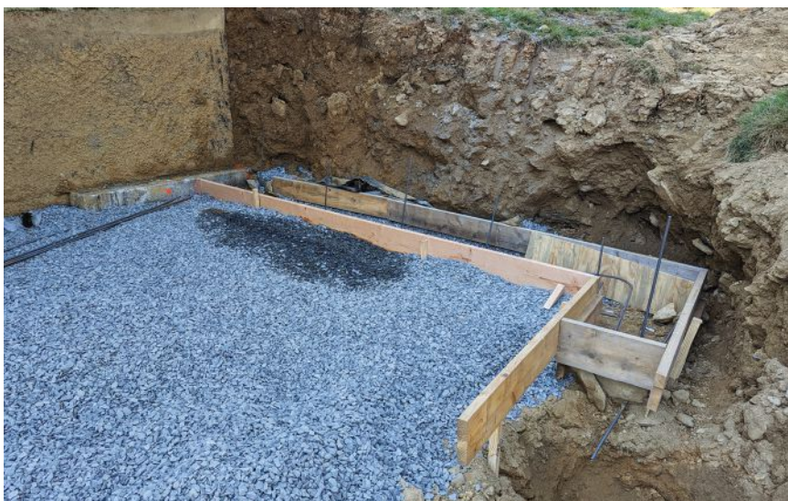
Shown here is the formwork for the footings that will support an engineered block retaining wall needed to partially enclose a dry storage area underneath the deck.
