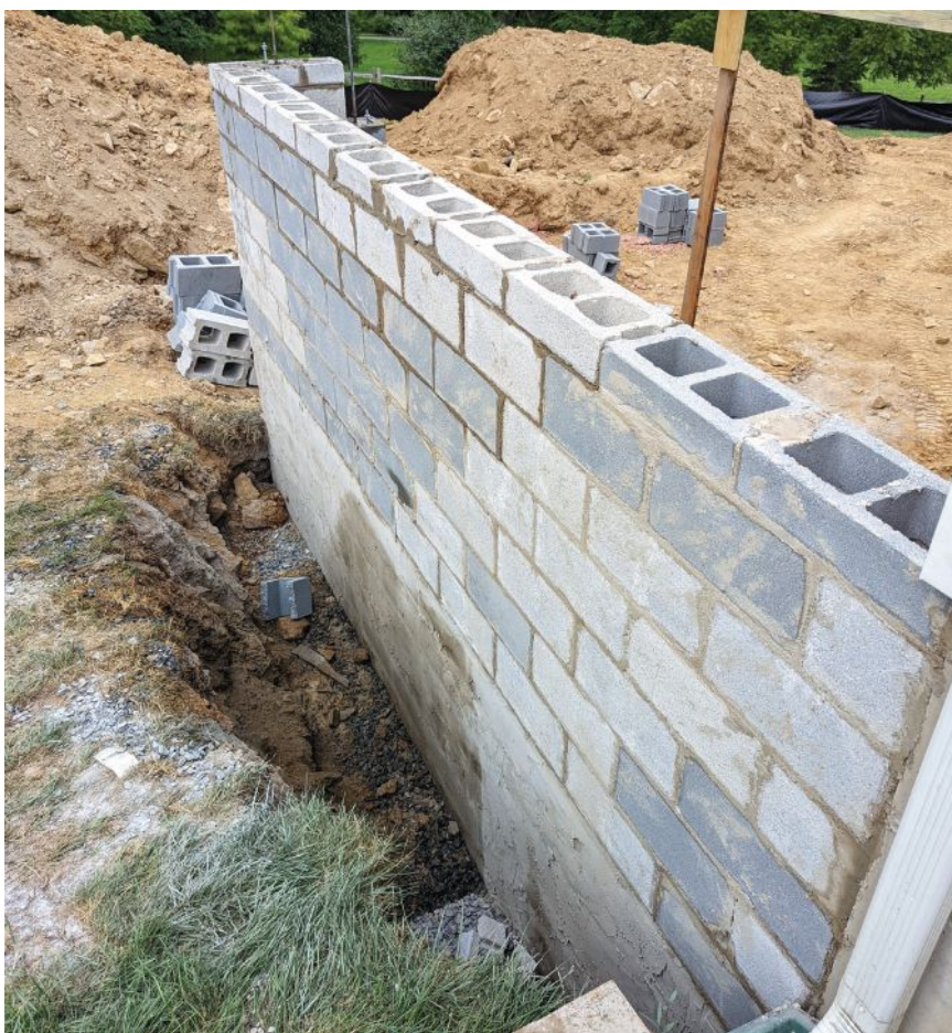
Here, the block retaining wall is under construction. To reinforce the wall, the cores will be filled with concrete and rebar.
