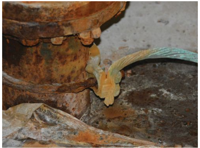
Red flags, from left to right: A bond wire is cut between two pumps; and a corroded ground electrode connection spells a hazard.
