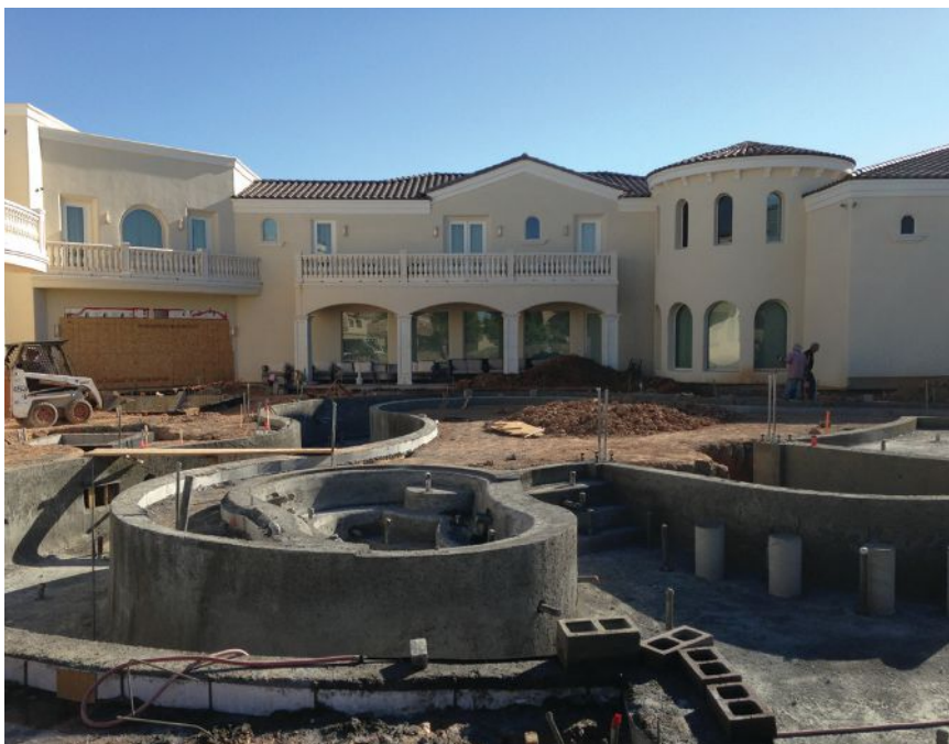
Soil conditions may be a concern in one respect: Because lazy rivers cover more ground than most pools and spas, there is increased risk of differential soil conditions, which could lead to uneven settling. Builders and designers should seek the counsel of soils engineers.
