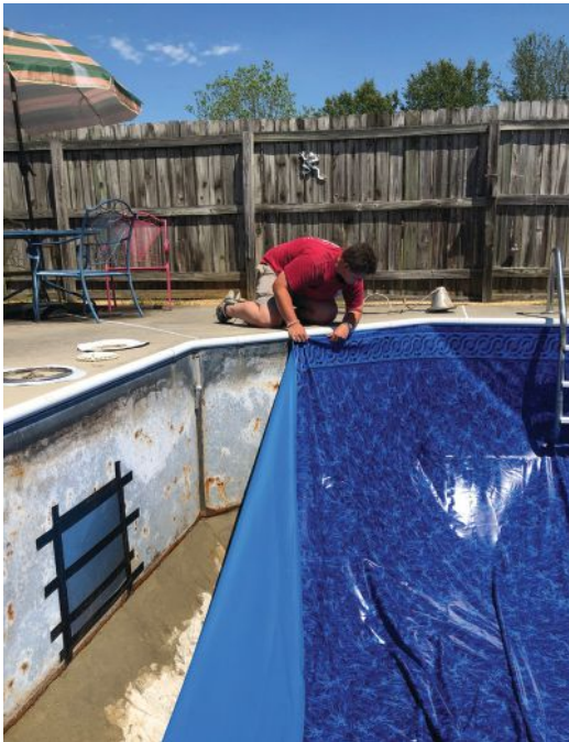
Try to prolong ordering the liner until after the excavation and installation of the panels.
