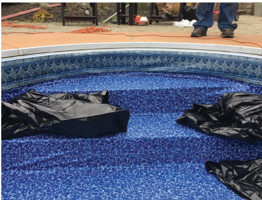
Weighing down steps, benches and other special features can help secure them in place while the liner is stretched in place.
