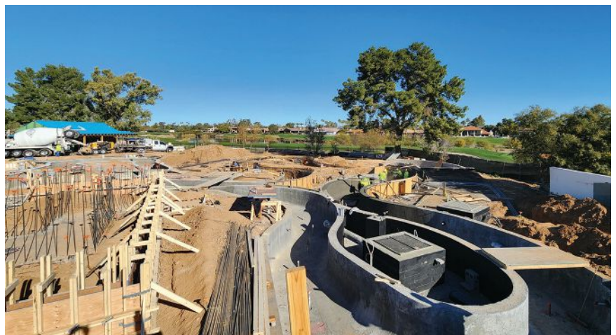
Various stages of the lazy river. At the bottom, the shotcrete is extended across one of the river's loops to strengthen the structure.
