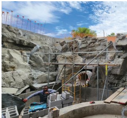
The artificial rock will be used throughout the grotto and slide area.
