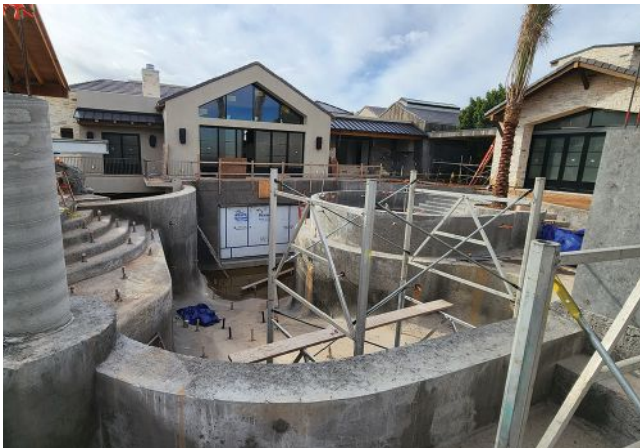
Clockwise, beginning top left: The palm trees were set in place early in the process, when access was more clear. The pavilion and swim-up bar make progress. The main pool is seen from another angle. An intricate shoring system is used to support forms for the grotto deck.
