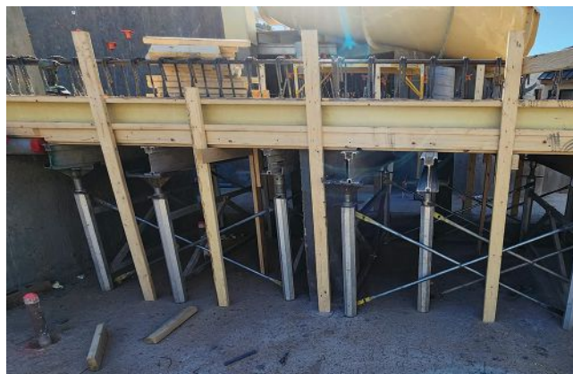
Clockwise from top left: Floating stainless steel stairs leading into a lower catch basin. Shoring for the roof of the grotto. The pool that will house the FlowRider surf simulator. Shoring and forming for the bridge between the river and surf simulator intake.
