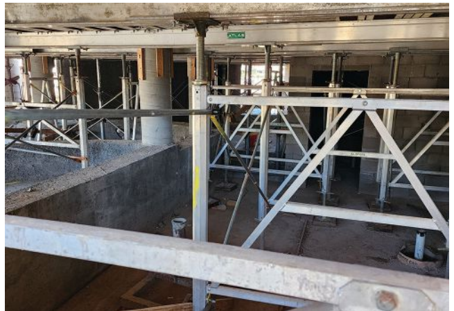
Clockwise, beginning top left: The palm trees were set in place early in the process, when access was more clear. The pavilion and swim-up bar make progress. The main pool is seen from another angle. An intricate shoring system is used to support forms for the grotto deck.
