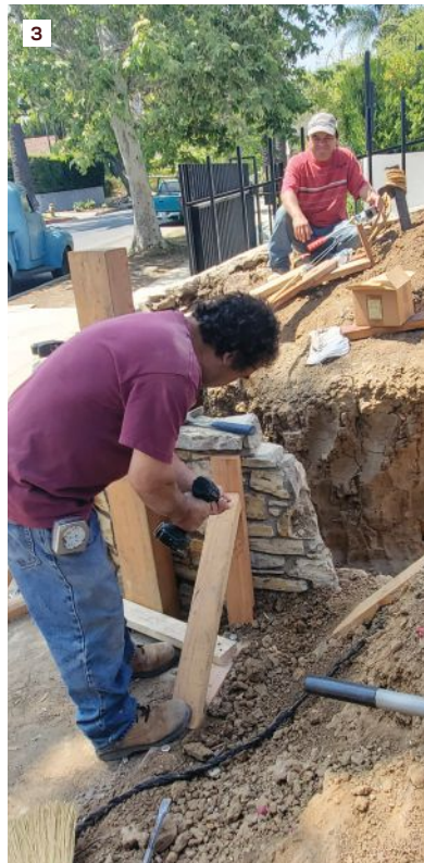
At the street-adjacent curved section of wall, a steel anchor post was driven into undisturbed soil (2). A come-along attached to the steel anchor and a 4-by wall brace pulled the wall back to plumb. Workers reset the 2x4 angled bracing after plumbing up the wall (3).
