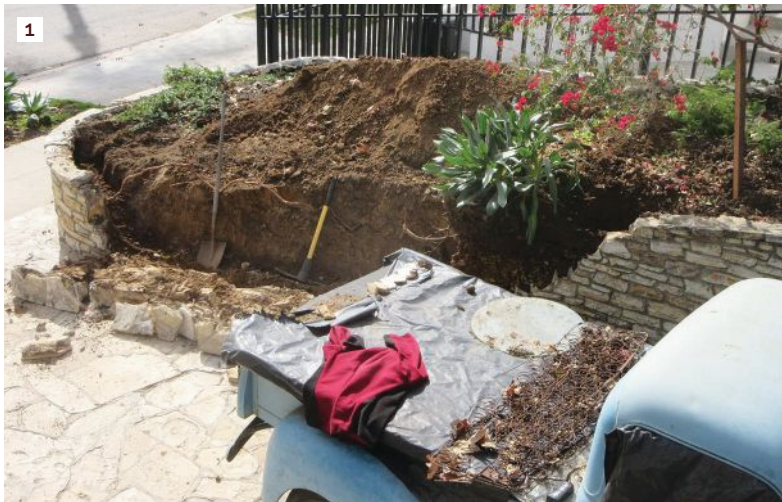
The middle third of a leaning, unreinforced stone retaining wall collapsed during excavation by the homeowner (1).
