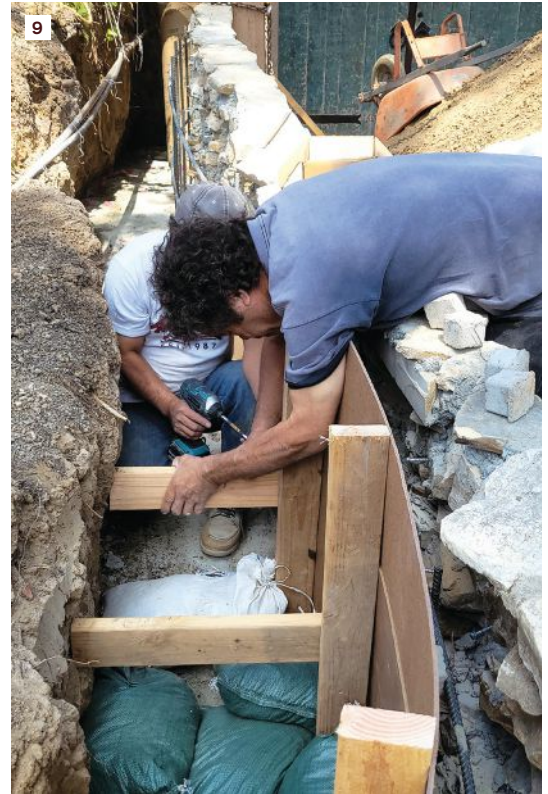
The collapsed portion of the wall was rebuilt using salvaged and new stone (8). Sheets of 1/4-inch-thick Masonite, 2x4 horizontal blocks, and sandbags were used as wall forms on the shorter curved wall sections (9).
