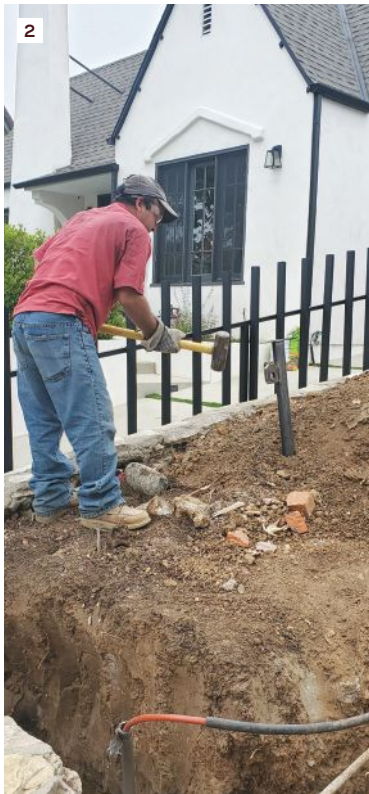
At the street-adjacent curved section of wall, a steel anchor post was driven into undisturbed soil (2). A come-along attached to the steel anchor and a 4-by wall brace pulled the wall back to plumb. Workers reset the 2x4 angled bracing after plumbing up the wall (3).
