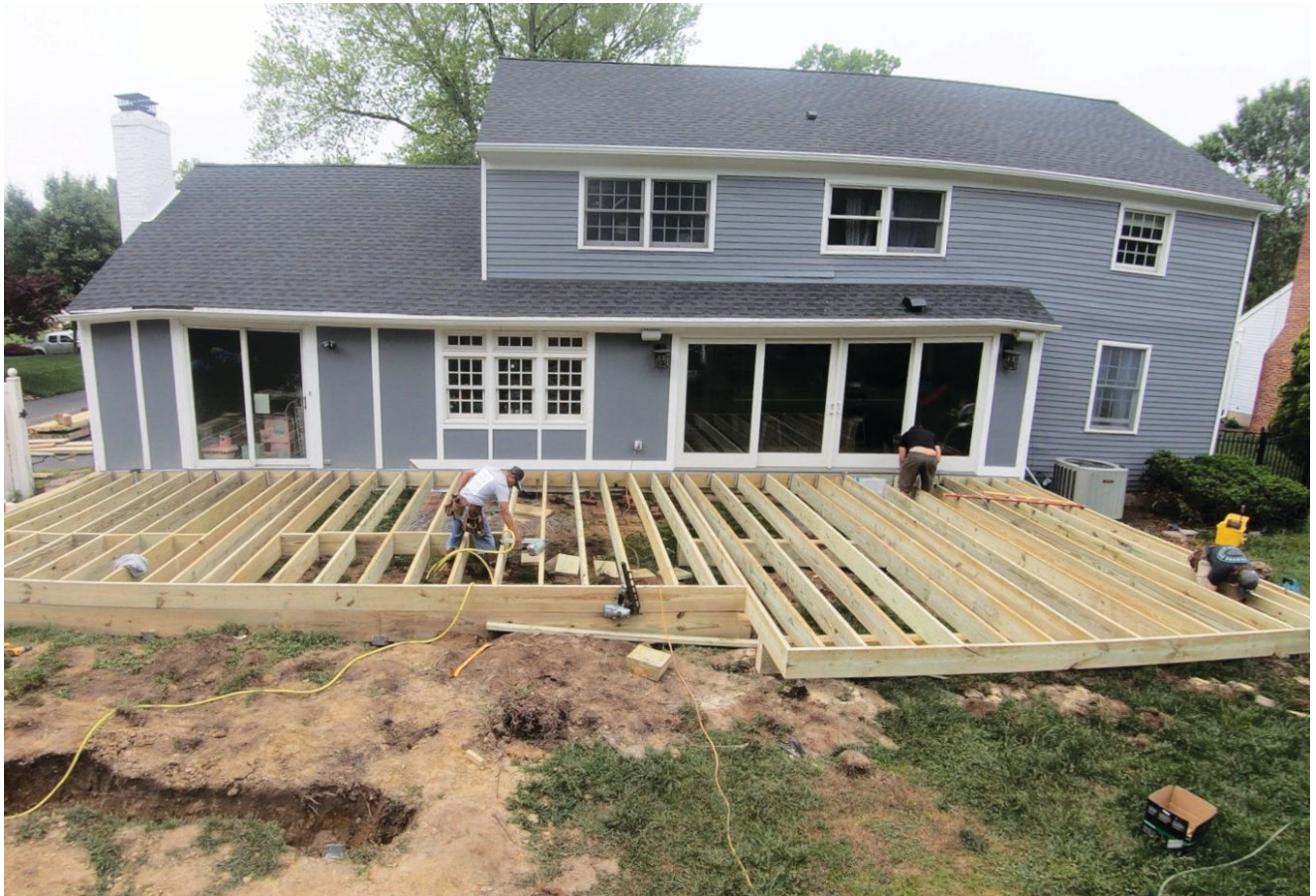
Most of the deck was conventionally framed with pressure-treated lumber.
