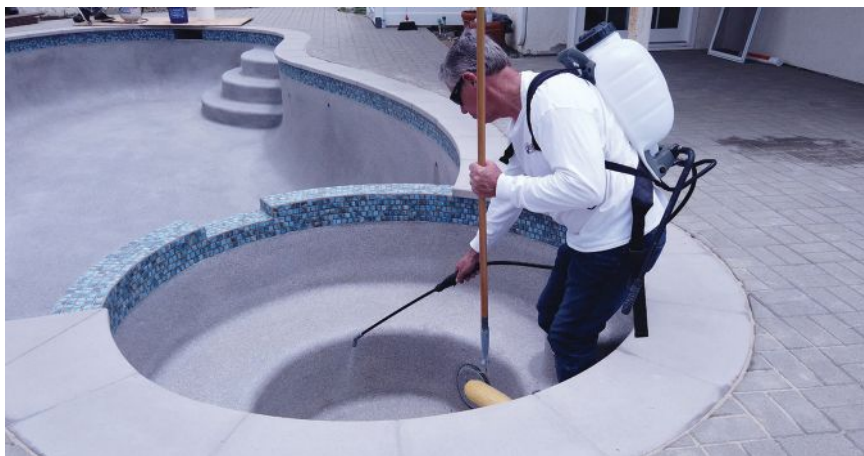
MicroGlass is applied with a backpack sprayer in one to two coats onto plaster, pebble and other cementitious finishes. It can be applied to newly applied or older surfaces.
