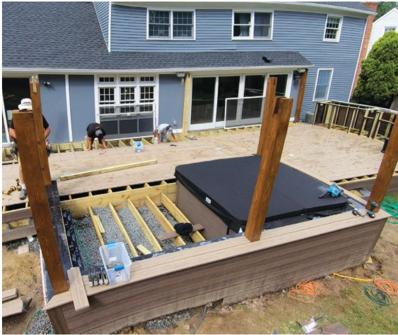
6x6 posts were added to the design to provide support for simple, single-ply beams that support overhead lighting and a deck-cooling misting system.
