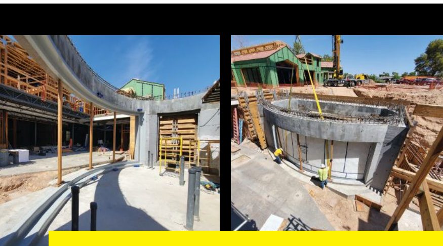
The shark tank is erected before contractors build the basement room in which it will sit. The radiused acrylic panel that provides most of the viewing measures 350 inches wide and 130 inches tall. It had to be ordered well in advance, so the team had to build the structure and rebates precisely to fit the sizable piece.
