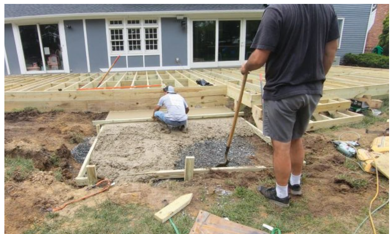
Workers poured a slab to support the hot tub.
