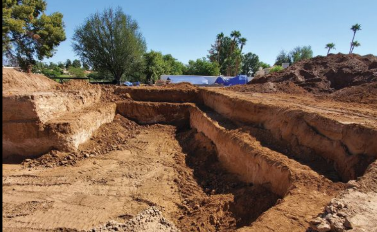
Left: The basement pool in progress. The rock waterfall is being built one terrace at a time. Right: crews begin excavation for the go-kart track, which begins on grade, then dips underground.
