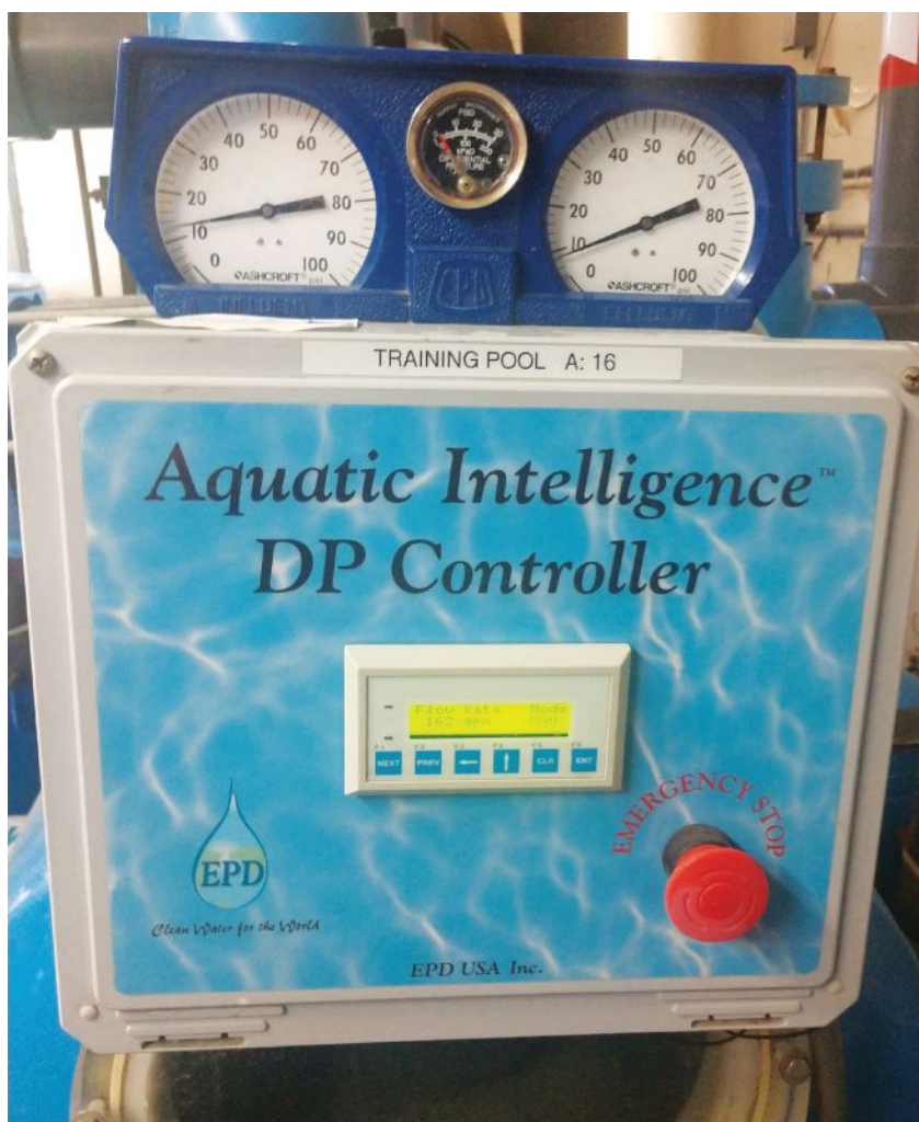
It's best to use a combination of interlocks to prevent chlorine gas incidents.
