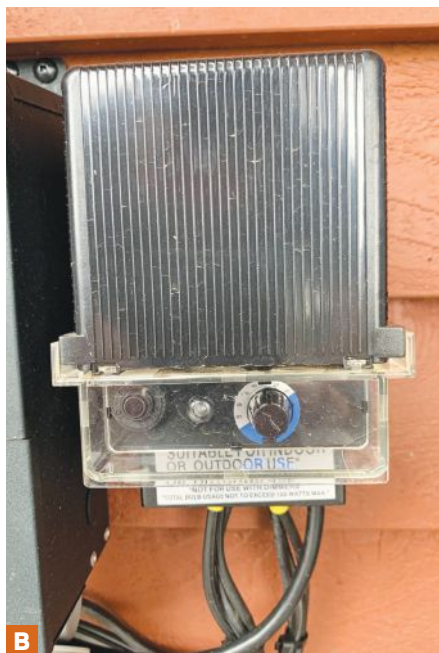
Figure 1. Most LED lighting systems can be powered by a 12-volt DC transformer, but some systems are designed to operate at 24 volts DC (A). This 24-volt DC unit has an external programmable photoelectric sensor (B).
