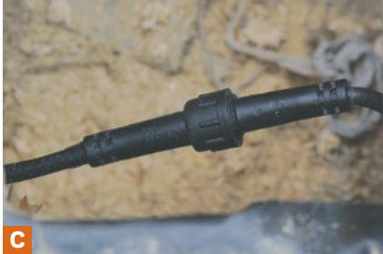
Figure 2. Low-voltage two-wire cable is UV-protected and weatherproof, so it doesn't have to be run in conduit (A). While there is no industry standard for fittings, companies such as In-Lite offer high-quality waterproof cable connectors for extending lines (B, C), connecting fixtures to supply lines, and adding branch lines (D).
