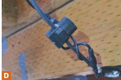
Figure 2. Low-voltage two-wire cable is UV-protected and weatherproof, so it doesn't have to be run in conduit (A). While there is no industry standard for fittings, companies such as In-Lite offer high-quality waterproof cable connectors for extending lines (B, C), connecting fixtures to supply lines, and adding branch lines (D).
