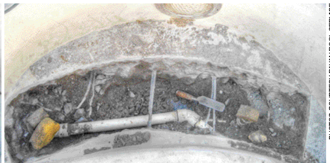
The big fake-out: At first, this system appeared legitimate, above left. Each drain had two pipes — one presumably connecting to the pump and the other to the skimmer equalization line. But when air was forced through the skimmer, bubbles only came out of one drain. Professionals cut the concrete to investigate, above right. But the drains ran separately. The two stub-ups with connecting pipe, opposite, led to nowhere, and seemed to be just for show.
