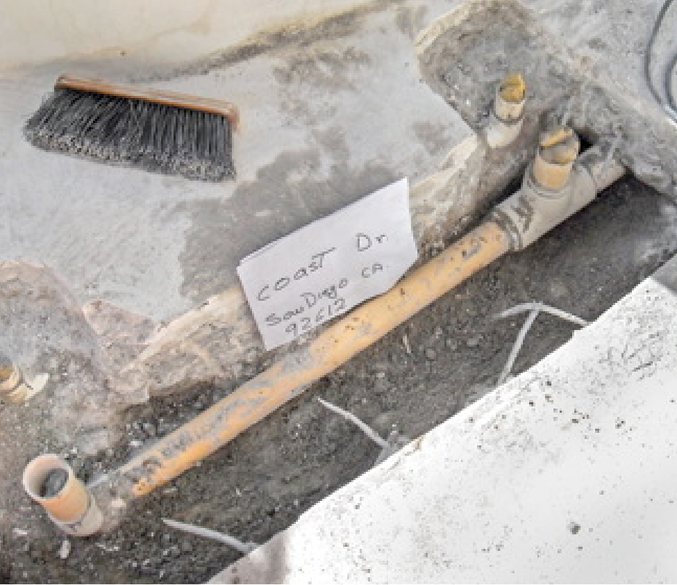
The right and wrong way: Service professional Javier Payan photographs each drain configuration he inspects, with the address included in the frame. In the top photo, the drains are not balanced, with the tee sitting below the right outlet. Cutting pipes on another site, middle, shows they are clogged with concrete, rendering one of the drains useless. At bottom, a properly re-plumbed dual-drain system, with the tee set in the middle.
